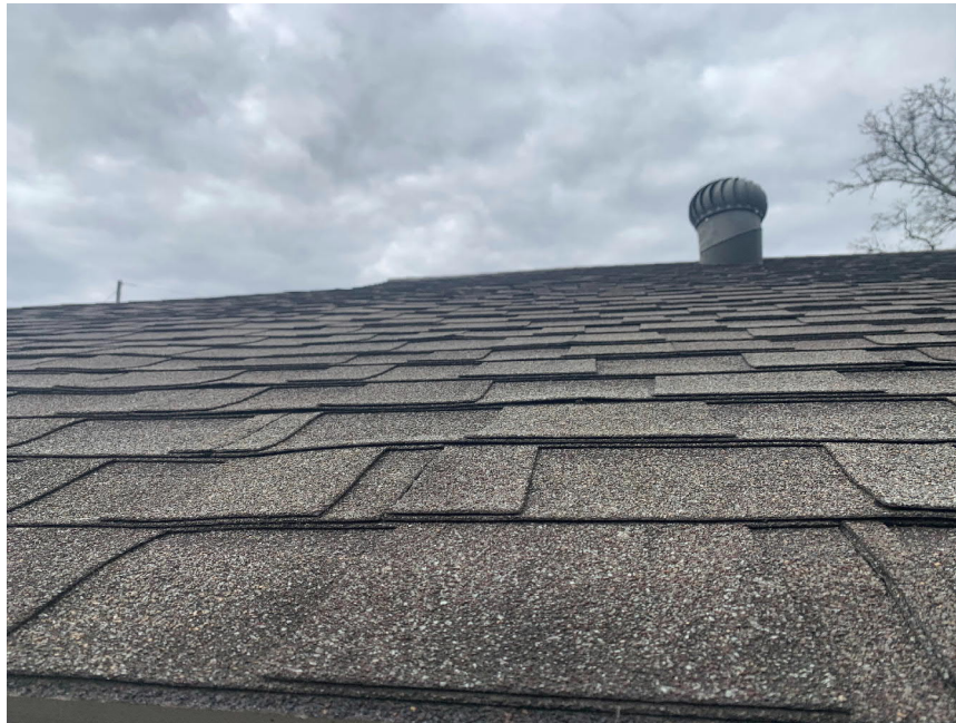
Photograph No. 5 HA-05: Black Roof Shingles with Black Tar Paper
